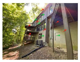
The painting project will include powerwashing and preparation (scraping, repair, caulking, etc.) of the areas to be painted and the application of two coats of Sherwin-Williams Intellectual Gray color paint to the block, fascia, siding, and soffit.
